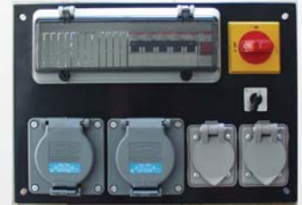
8kVA Generator option available on M64.
