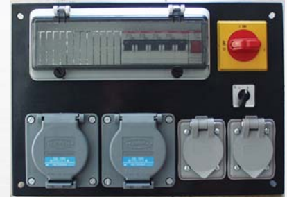
8kVA Generator option available on M100.
